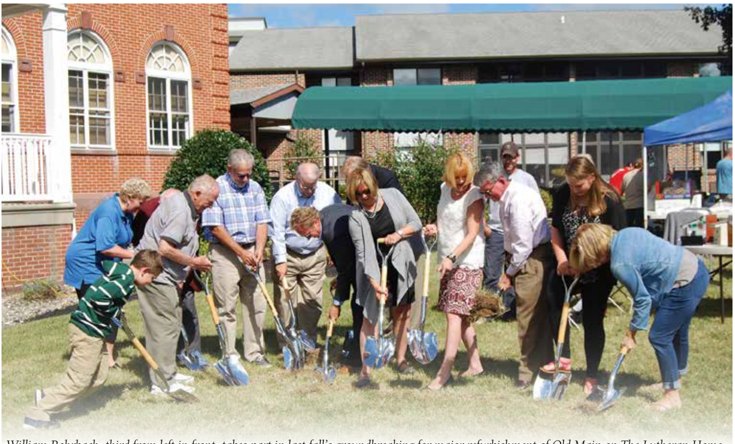
William Rohrbach, third from left in front, takes part in last fall's groundbreaking for major refurbishment of Old Main on The Lutheran Home at Tipton campus. The project will create a permanency center in Old Main related to adoption and foster care—a direct connection to the initial children's services at the home that once benefited Rohrbach.
