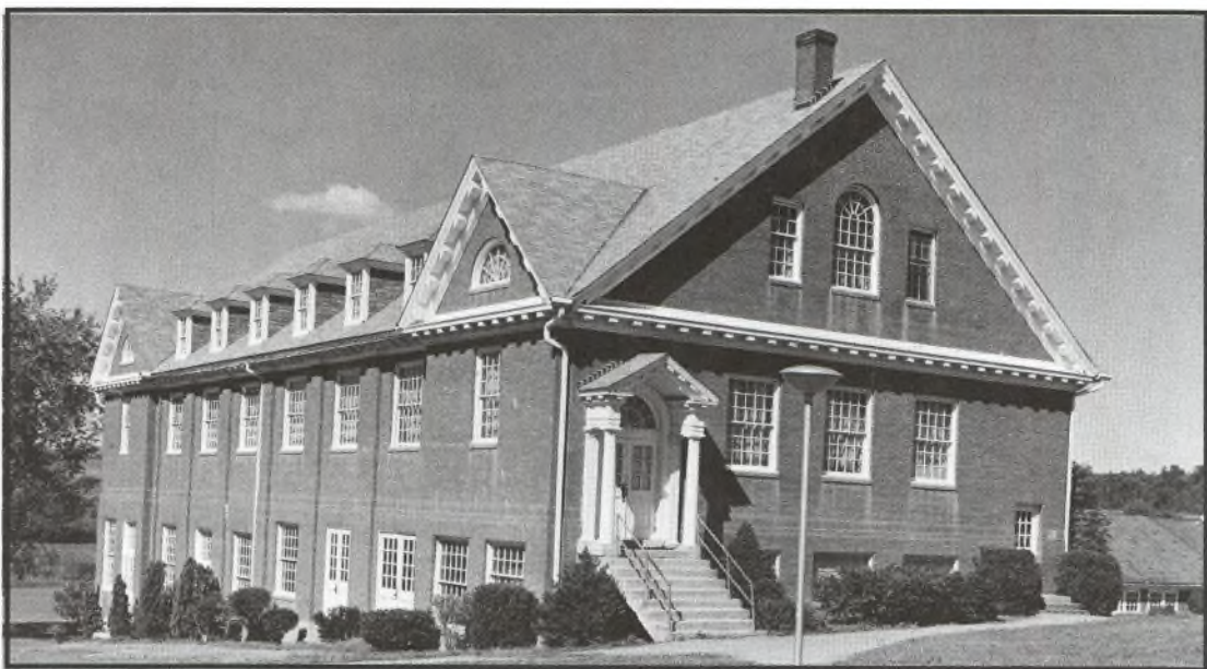
(Top) A class at the plumbing shop in the home's Charles A. Widle Trade School, dedicated in June 1926. The instructor, at left, is Theodore Allison, the home's chief plumber. (Bottom) The trade school building, which also contained a gymnasium.
