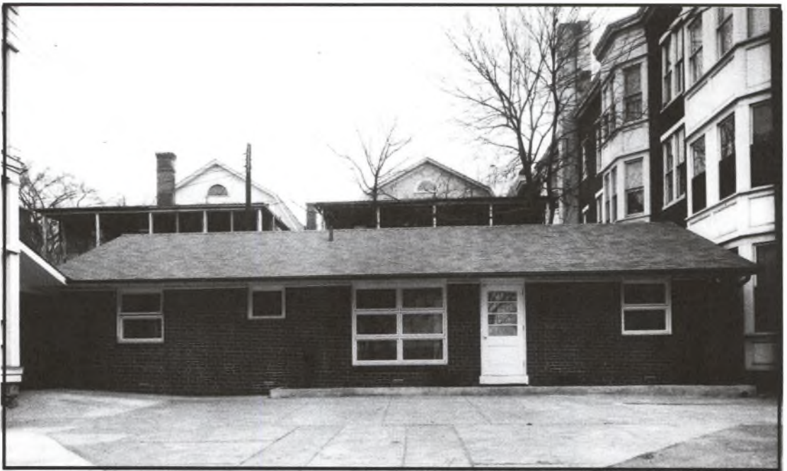
The "cottage" constructed adjacent to the Harrisburg home.
