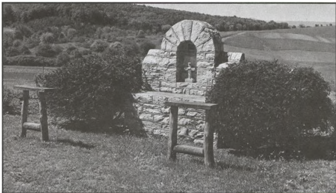
During the summers of 1943 and 1944, older boys at the home constructed a hillside altar for use in outdoor worship services.
